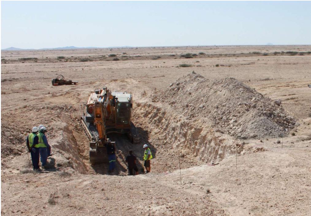
Figure 4 Excavation of Test Pit at Marenica
